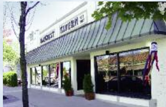
OAKCREST TAVERN 4022 N. OAKLAND AVE. Improvements include a new door and windows.
