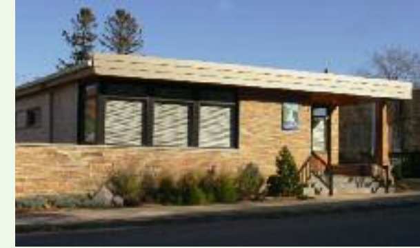
OFFICES OF TIMOTHY HART, D.D.S AND DR. JESSE SMITH, D.D.S. 1729 E. LAKE BLUFF BLVD. Improvements include new brickwork, windows and landscaping.
