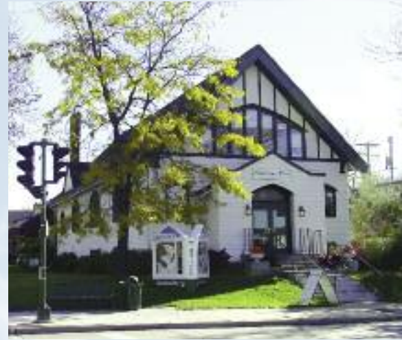
SHOREWOOD PRESS/ROBERT LAURENCE SALON 4060 N. OAKLAND AVE. Improvements include new siding, windows and doors.
