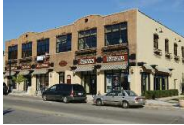
3510 N. OAKLAND AVE. Improvements include new windows, signage and decorative ironwork.
